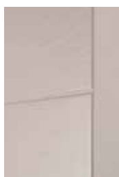
Particolare fresatura Close-up of machined groove
